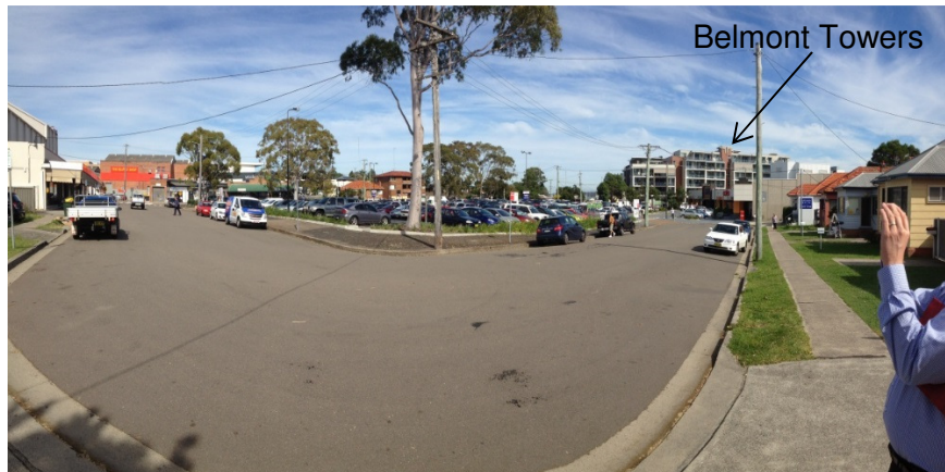
Figure 3-19: Eastern End of Coles Car Park Looking West
